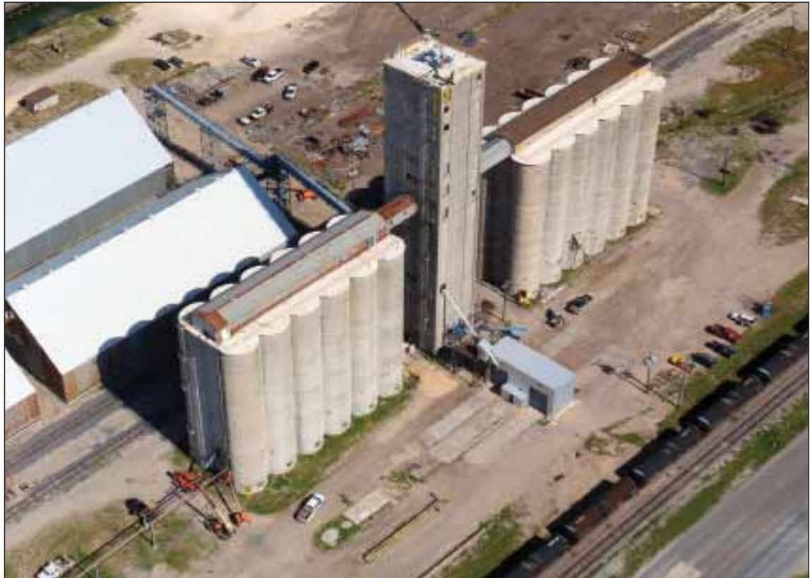
The port terminal elevator at Brownsville, TX, built in the 1960s and mothballed since 2010, has been refurbished by West Plains LLC and was scheduled to reopen partially on Feb. 1. Photos by Ed Zdrojewski.
